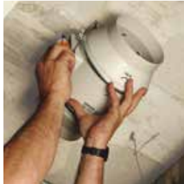
Place the impeller and motor assembly.
