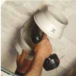
Fix the support bracket.
